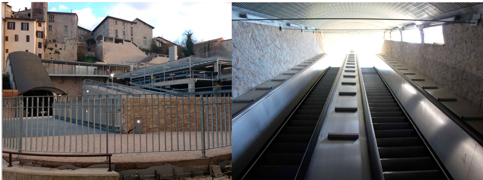
Figure 6. First extract: cost of the work: 33,5 million €. Functional composition: Parking 'Posterna' with a capacity of 450 vehicles (underground park multi-storey); mechanised path Parking 'Posterna-Piazza Campello' (underground with 7 couples of tapis-roulant); 4 elevators exit; mechanised path Parking 'Posterna', 2 elevators exit and 2 pedestrian exits.
